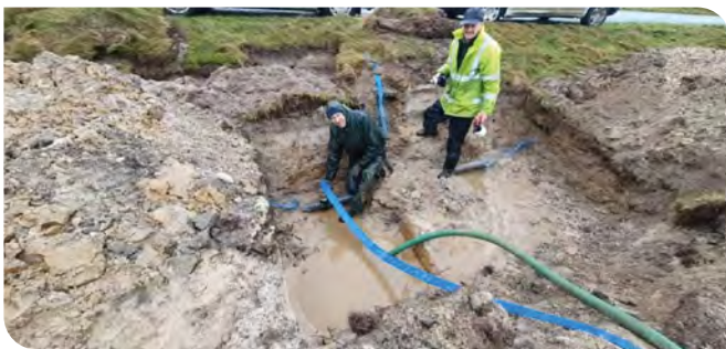
In total, it took around eight months to install the network
